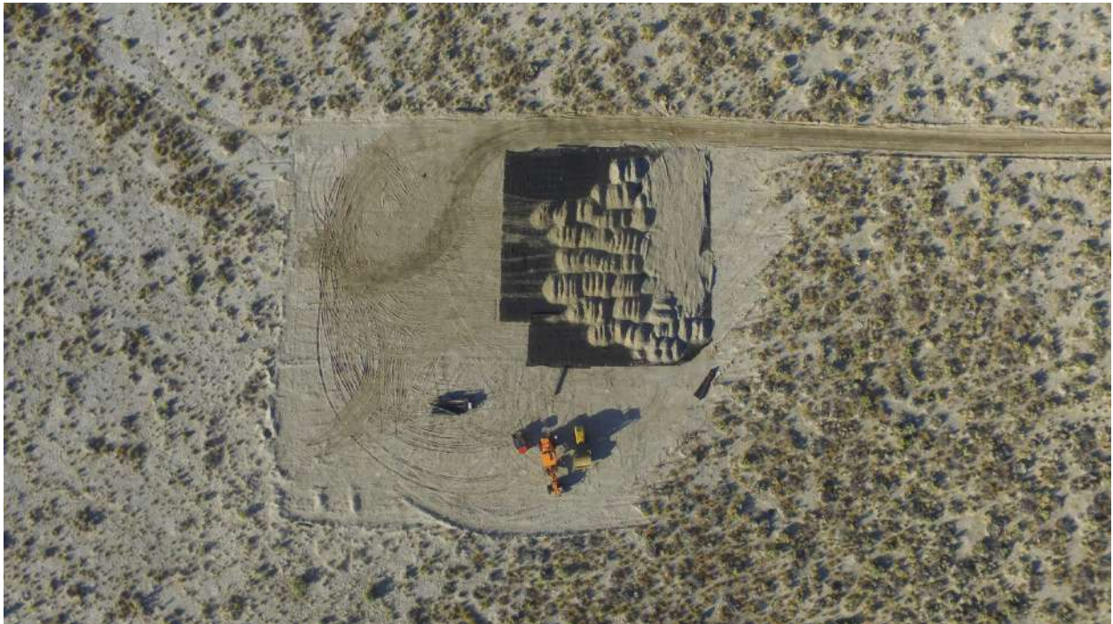
Figure 9-3 Drill Pad DH-2 Under Construction – from above
