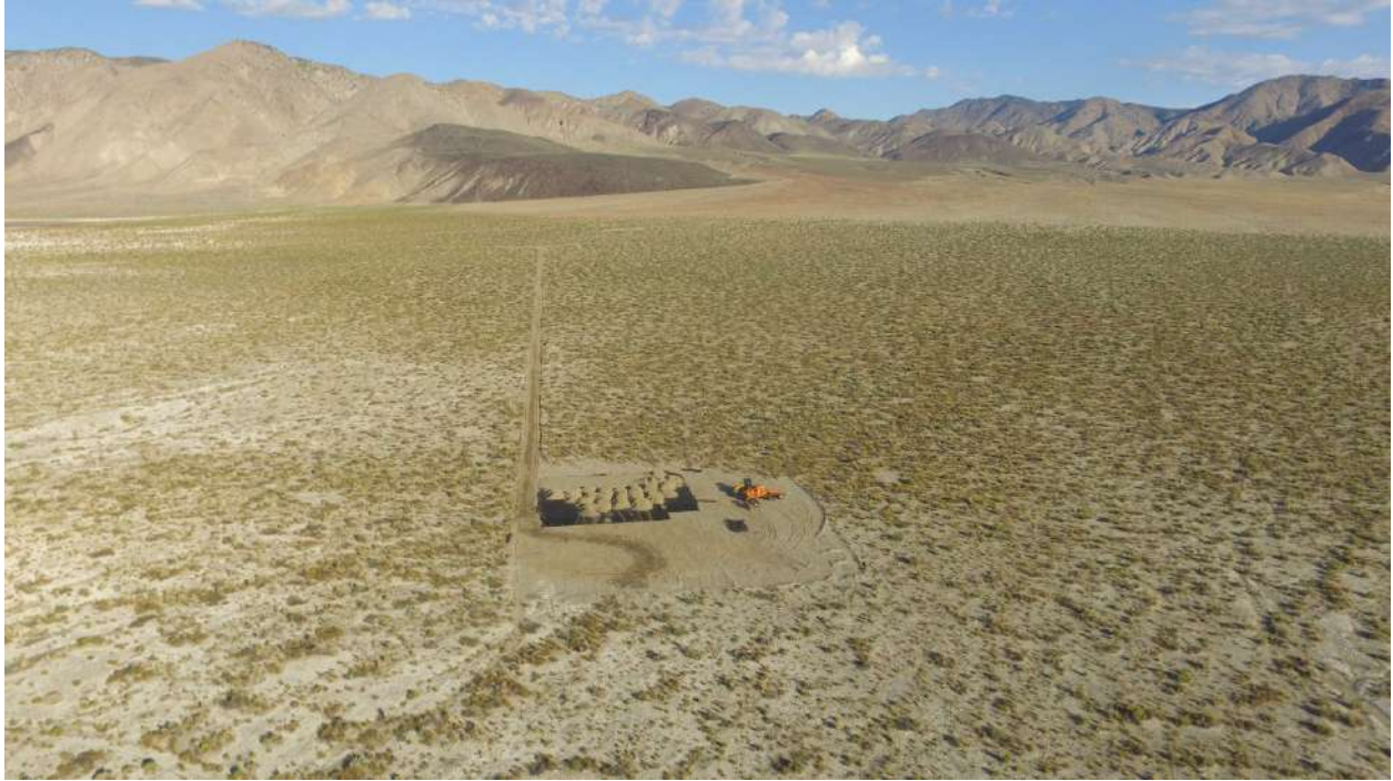
Figure 9-2 Drill Pad DH-2 Under Construction – looking west
