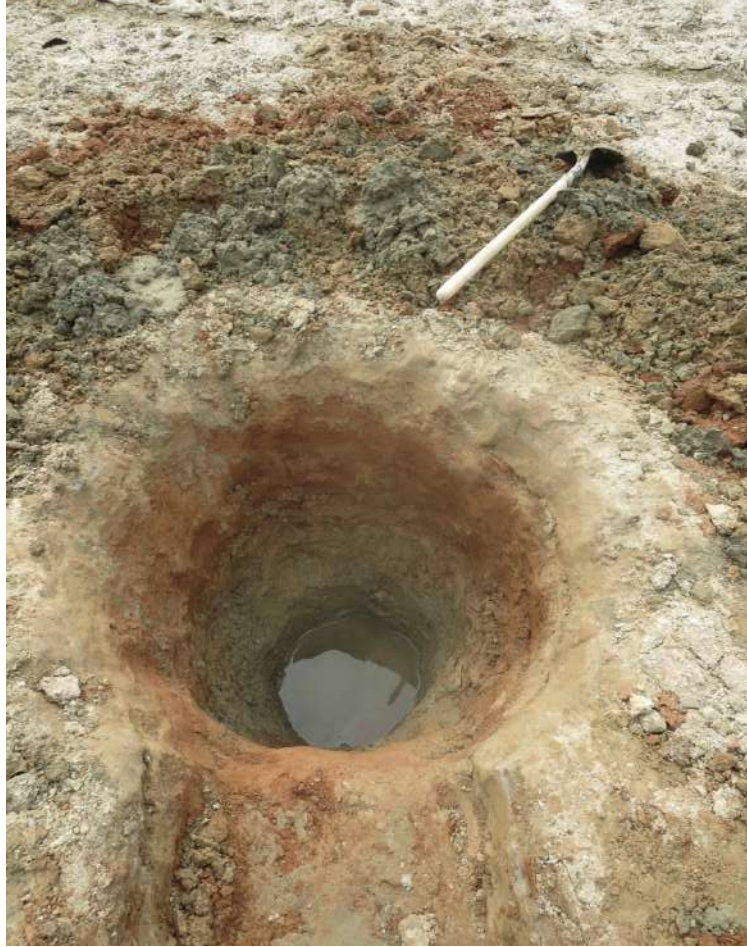
Figure 9-6 Completed brine pit at Site T-25 Sept 2020
