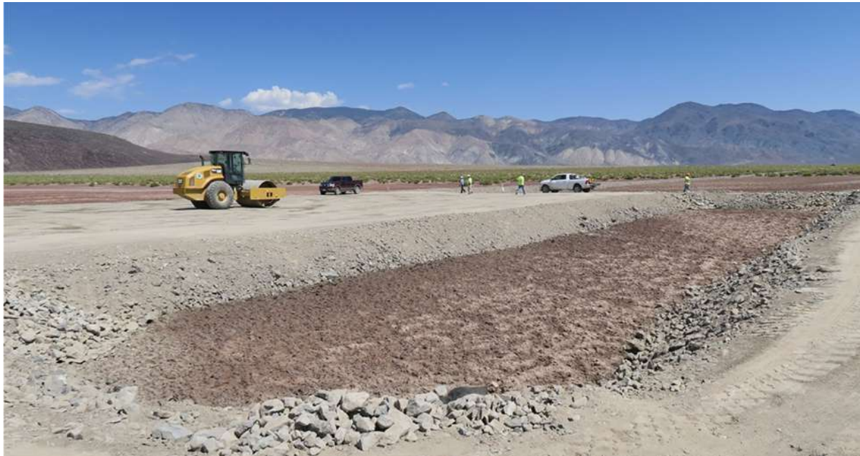
Figure 9-4 Constructed Drill Pad and Sump
